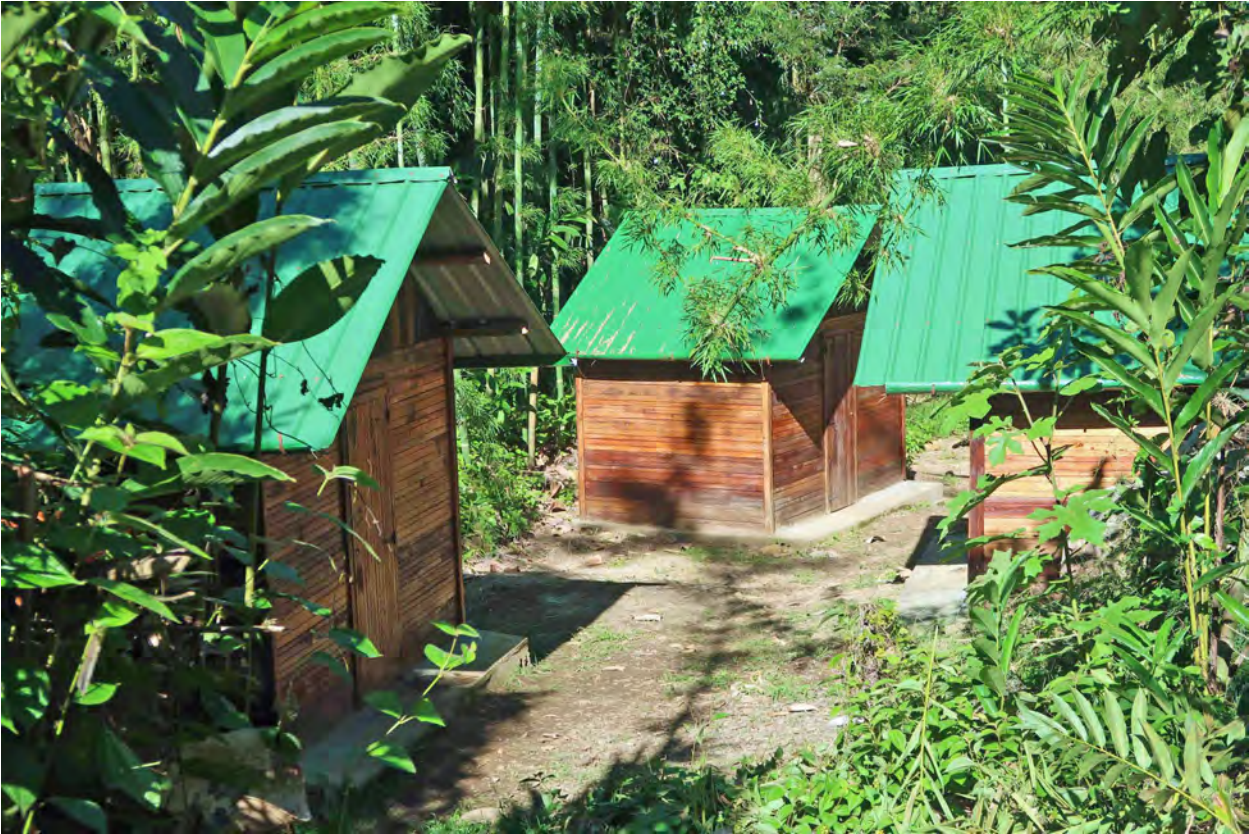
Figure 2. To enhance the visits of ecotourists at Marojejy, some infrastructure has been built over the past years along the Mandena-summit trail, including bungalows, cooking and eating structures, and sanitary facilities. After the recent passage of a cyclone in northeastern Madagascar, which impacted the Parc National de Marojejy, the previously built bungalows were severely damaged. With funding from Lemur Conservation Foundation, a considerable portion of the damaged infrastructure was rebuilt, such as the bungalows shown here at Camp Mantella at 450 m. (Photo by Erik Patel.)
